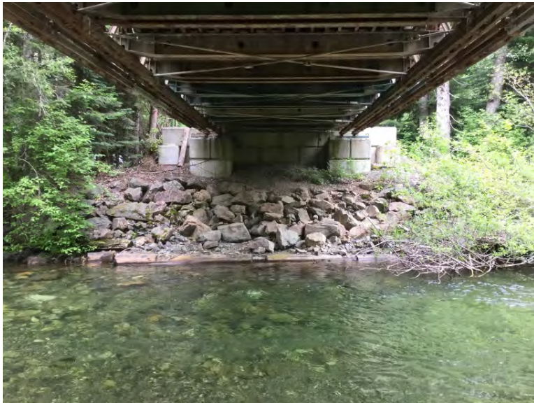
Right Bank Abutment when facing downstream
