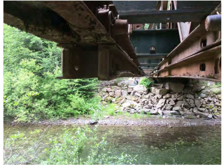
Up stream right bank chord condition
