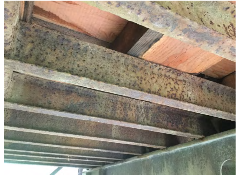
Bracing condition - typical
