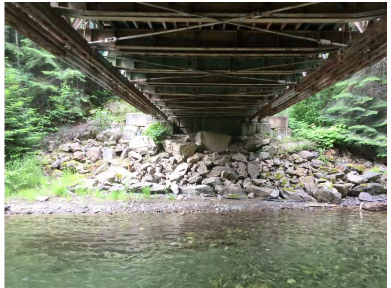
Left Bank Abutment when facing downstream
